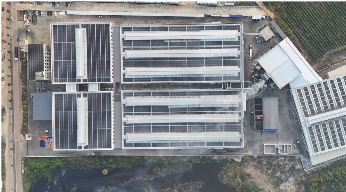
ZHONGXIN (THAILAND) 4.13 MW
